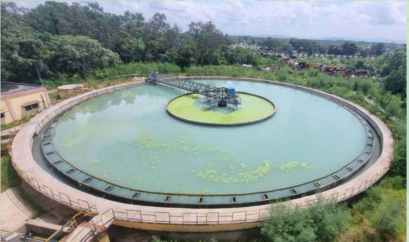
3000 M3/Hr CLARIFLOCCULATOR AT NALCO
